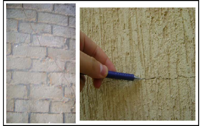
Fig. 2. Hair fractures at external wall of residential units at El-Rabwa Extension area.
